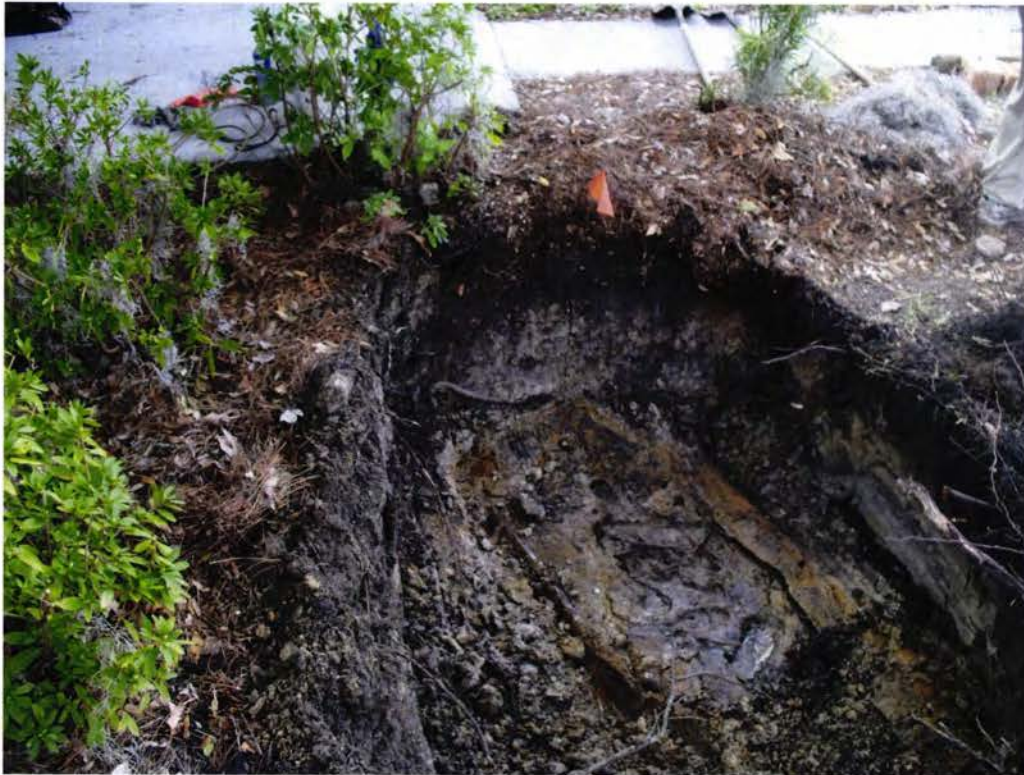
Picture 3: UST 257Beech-2 during excavation.
